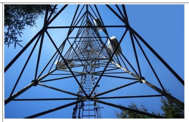
This telephone mast has triangular structures between the main poles.
